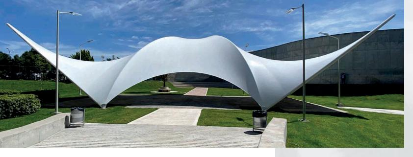
The cultural corridor design is characterized by the dynamism generated from the play and sequence of hyperbolic paraboloids, framed by metal structures with strategic points for the attachment of the **VALMEX**® FR 650-2 MEHATOP® F1 membrane, generating a greater visual impact and fulfilling the objective of providing protection to the 485 m² of the art corridor.
