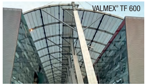
Shopping center roof
