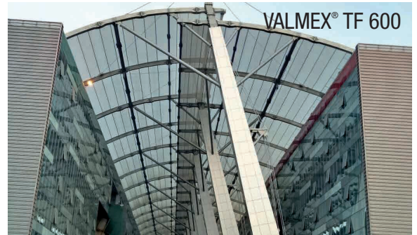
Shopping center roof
