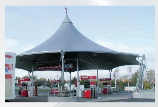
The gas station in Petersberg, too, has a canopy with a silver colour. It consists of one layer of Mehler Texnologies VALMEX® FR 1400 MEHATOP® F metallic Type IV.
