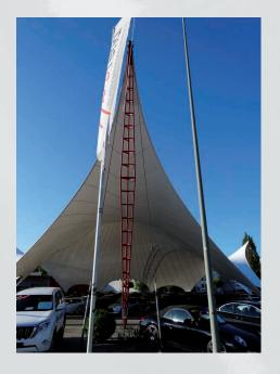
...HP Gasser AG was asked to refresh the construction by exchanging the membrane. A new VALMEX® FR 1000 MEHATOP® F Type III membrane was used to give the 20 year old building a mint look. The new material has similar material characteristics as the material used before, but adds with a new developed lacquering system a dash of 2017 technology to the construction. The advantages of the material used are high colour durability as well as shapestability combined with high tear resistance.
