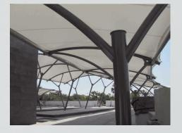
ding that the complete **VALMEX® FR 700** membranes had been pre-produced by Schafbock Design + Workshop. This took 45 days while the rest of the construction work was not disturbed during this period.
